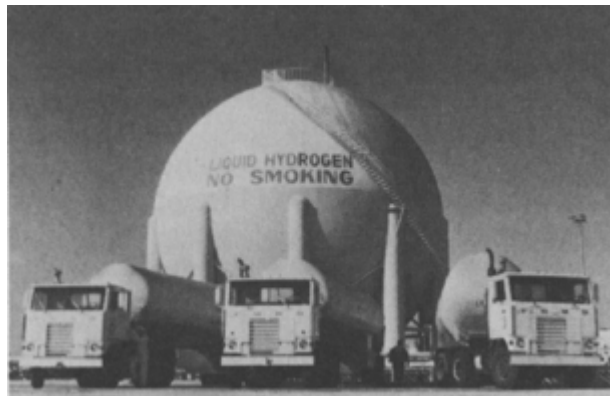
Abb. 35: 3800 m 3 LH 2 Speicher am Kennedy Space Flight Center in Florida (Photo NASA)
