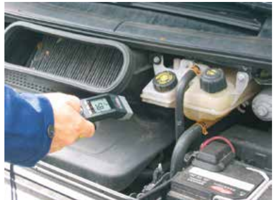
Checking the heating system
