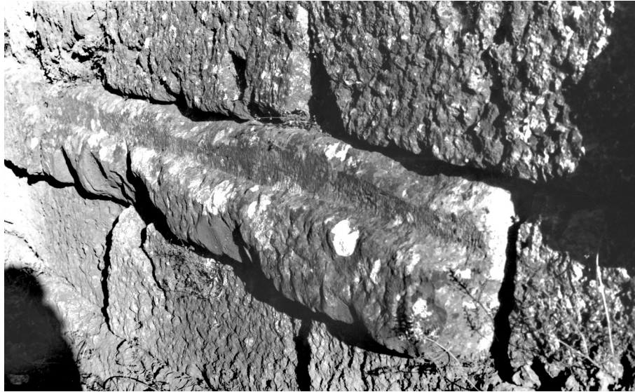
Figure 15. Marble block from the stylobate of the Early Archaic temple, reused as building material in the foundations of the Classical temple. (Photo: Østby)
