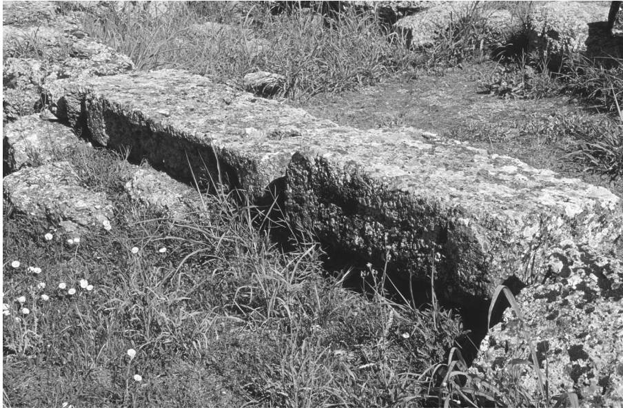
Figure 20. Two conglomerate blocks in the southern colonnade foundation of the Archaic temple. They have anathyrosis on the side surfaces, and were probably taken from an earlier building. (Photo: Østby)
