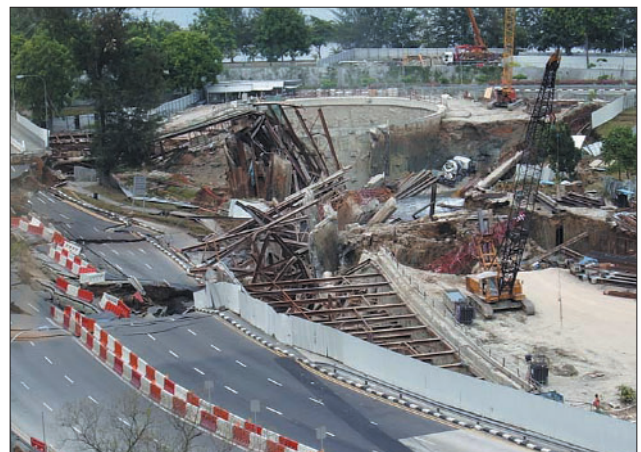
Abb. 1: Nicoll Highway Kollaps, Singapore
