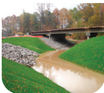
Houston USA, after installation
