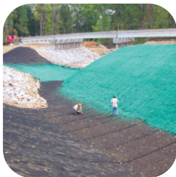
Houston USA, during installation
