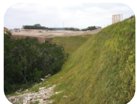
San Antonio USA, after installation
