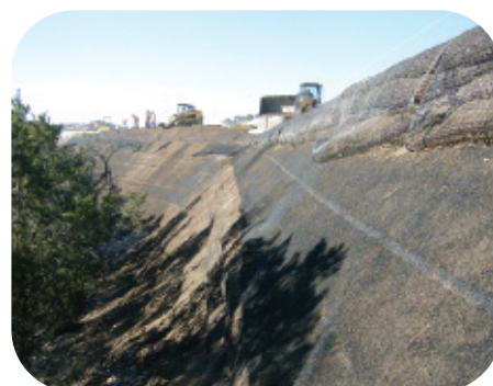
San Antonio USA, during installation
