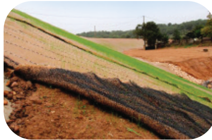
River dike protection against flooding Enkamat J Vauvert, France
