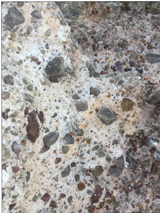
Fanglomerate exposure, PPL Landfill Cell 1A excavation, north side
