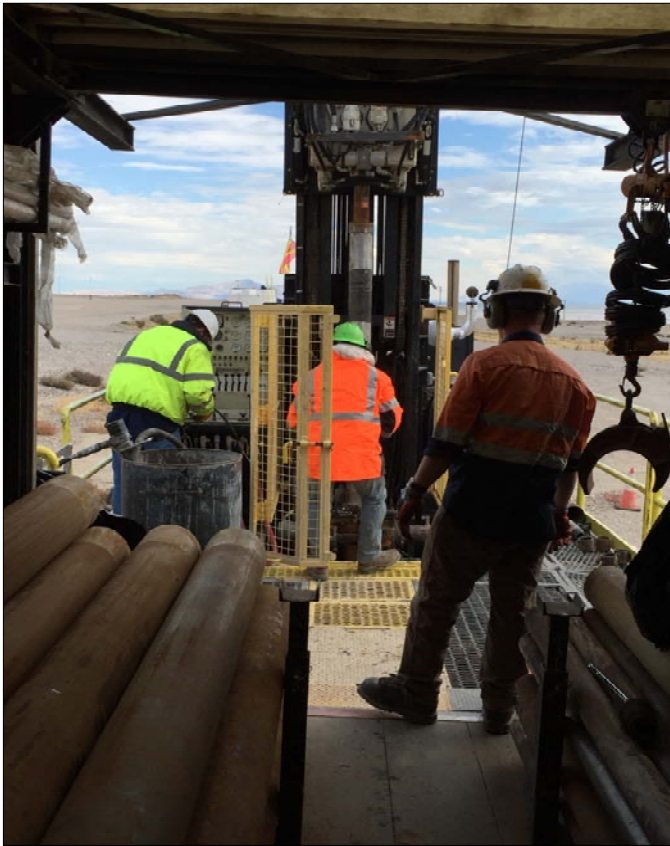
Running casing, sonic drilling boring MW-8
