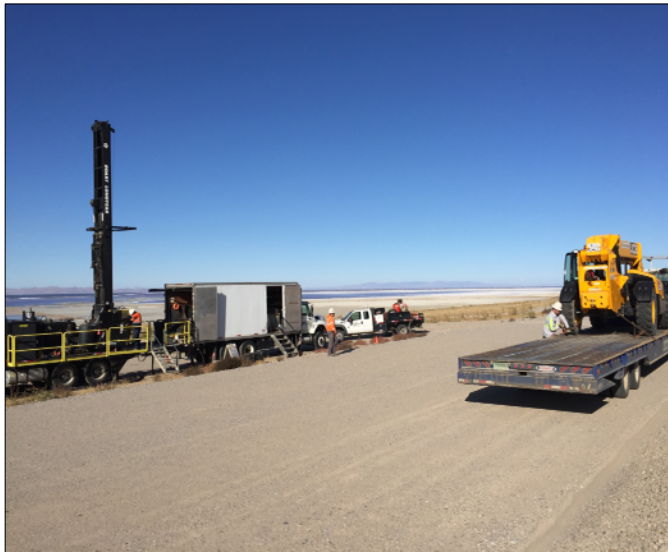
Drilling boring MW-8, looking west
