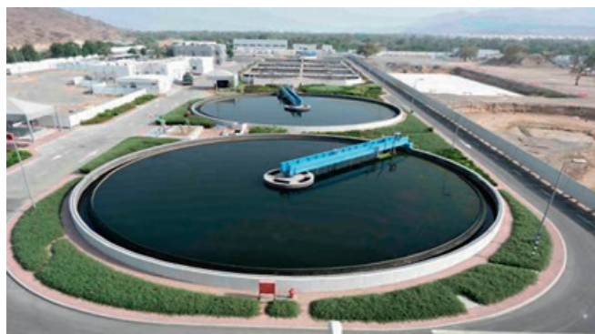
Fig. 1: Secondary Clarifier of the wastewater treatment plant of Fujairah, United Arab Emirates (UAE) (Photo: EW)
