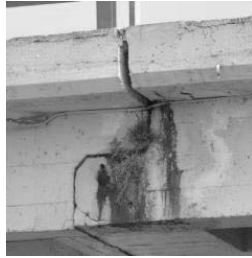
► Overpass road CV-500 (Valencia, Spain) © Mata-Falcón, Miguel, Pallarés, 2015
