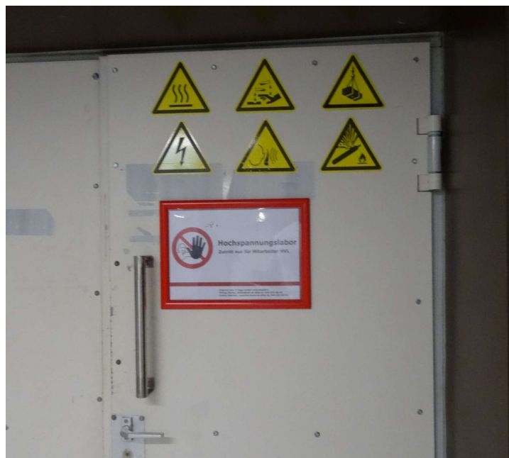
Figure 2: Example of Lab door signalment. Access restriction (red) and warning signs (yellow). Door Lab ETZ C79.
