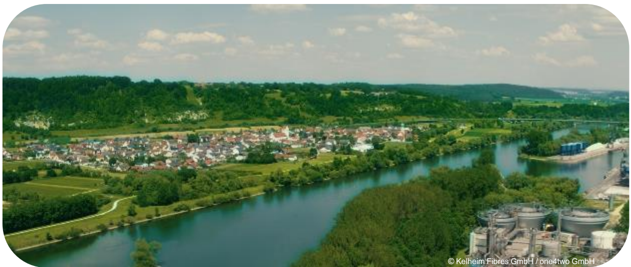
Biological waste water treatment plant: Our three vertical bioreactors in the Danube area
