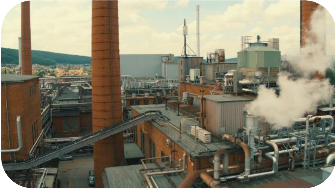
Our power plant
