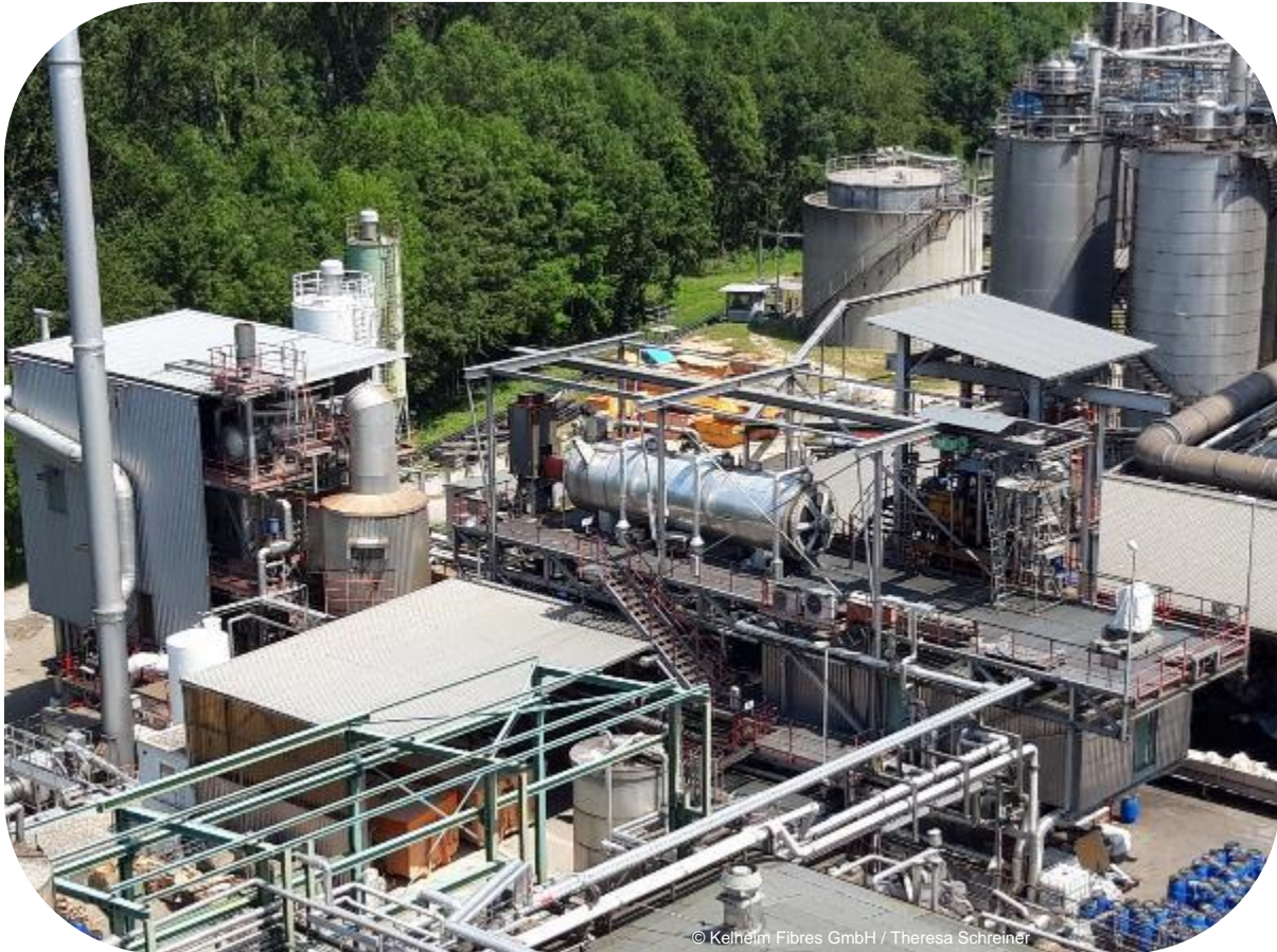
Area of the residue incineration plant
