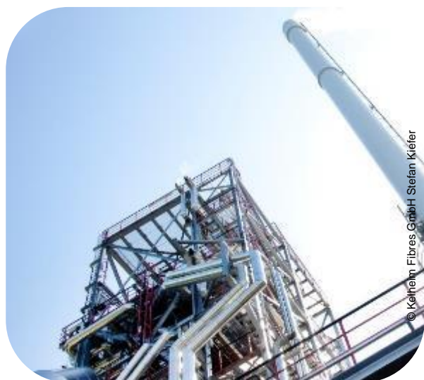
Sulphuric acid plant
