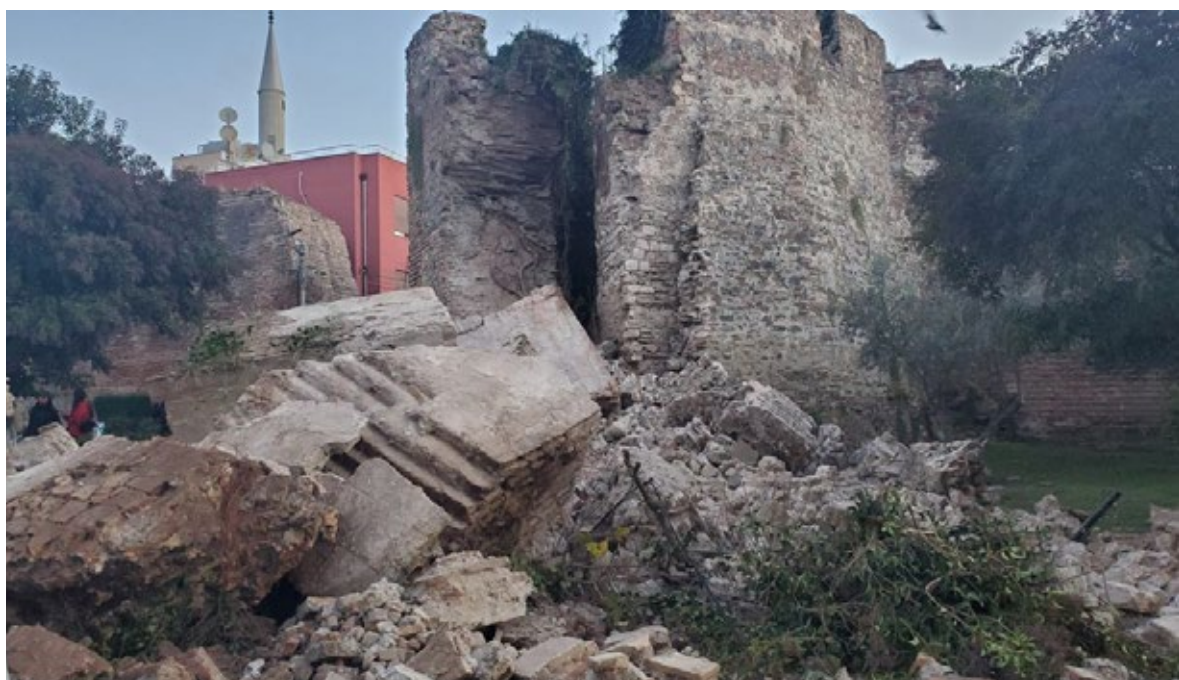
ANCIENT WALLS IN DURRËS, ALBANIA, DAMAGED BY THE EARTHQUAKE 2019
