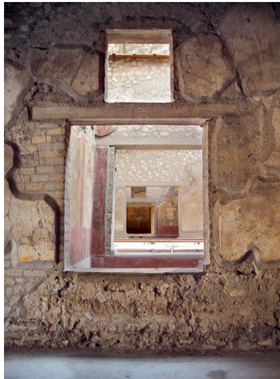
Fig. 7 Villa A at Torre Annunziata, view from room 73/74 through lightwell 70, room 69, lightwell 68 to room 64/65
