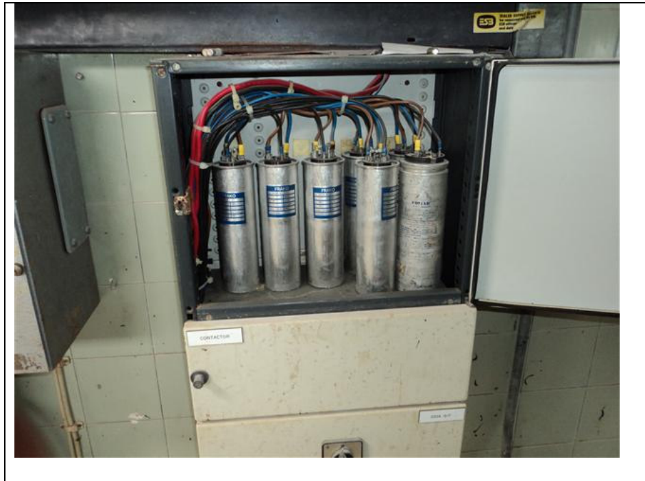
Image 7: Frako Capacitors which can contain PCBs (small cylinders in picture below)
