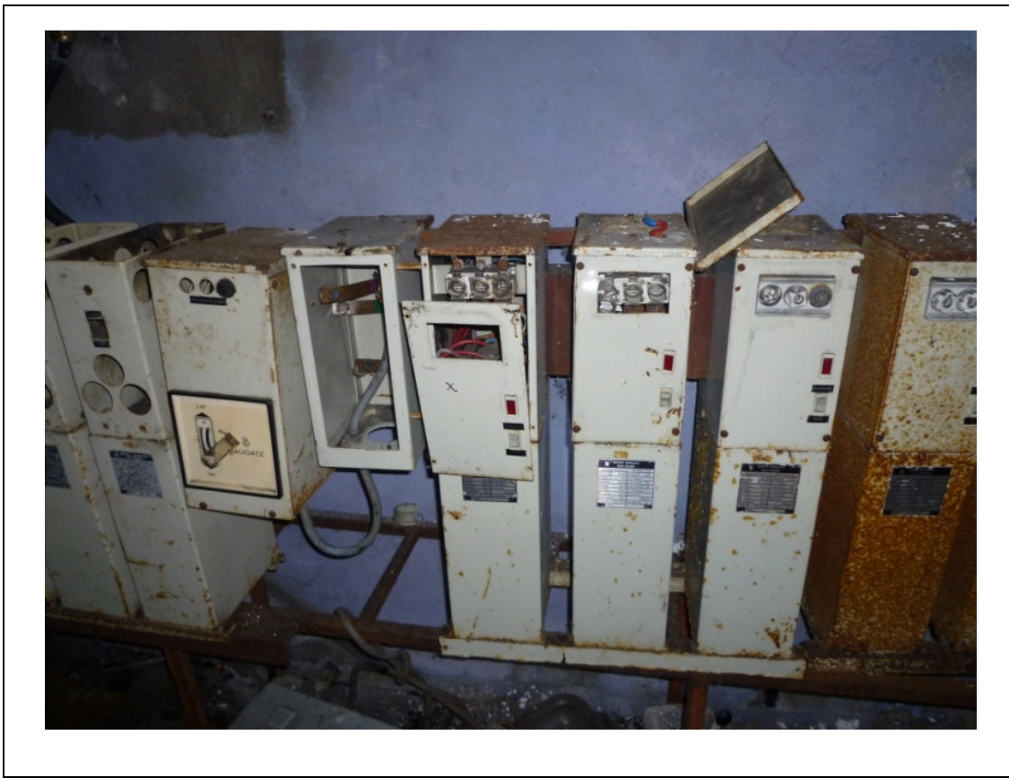
Image 5: Array of Baugatz capacitors (capacitors are the lower set of boxes below)
