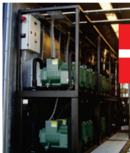
Frederikshavn, 1 MWq, CO 2 , heat delivery at 70°C, source: waste water, COP 3,1-3,4
