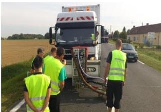
Orleans (South Paris), removal multilayer H.S.P./Paint from very soft SMA 800-1500 µ, full line
