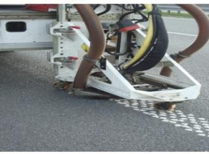
Gdynia, removal Thermoplastic Agglomerate
