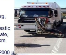
Kumla, removal Thermoplastic Full Line, from soft SMA, 2000 µ – 250 LM/hrs / + Agglo
