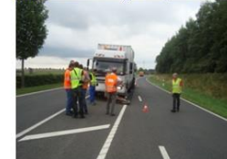
Luxemburg, removal Cold Plastic, Ribline from strong SMA, 10000/4000 µ
