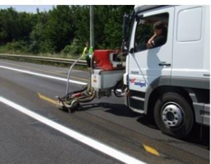
Battice, removal yellow HS paint from construction site, SMA, 600 µ
