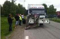
Jönköping, removal Thermoplastic Full
