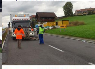
Emmen, removal Paint WB, Interrupted from poor SMA 300 µ
