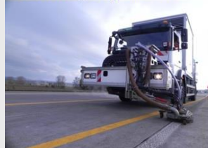
Eisenach, removal Cold Plastic Agglomerate from concrete, ~2000 µ
