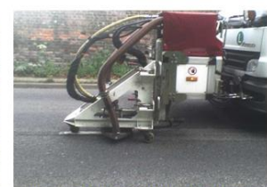
Oxford, removal Hot Spray Plastic, Full line, from poor SMA, 400 µ & Cambridge – removal Thermo Plastic, Hatches, from OPA 1000 µ
