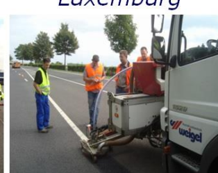
Luxemburg, removal Cold Plastic, Ribline from strong SMA, 10000/4000 µ
