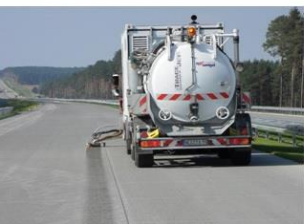
Rzepin (A2), removal Concrete film from concrete, 300 µ, full line
