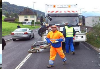
Emmen, removal Cold Plastic from very poor SMA, 1250 µ, full line
