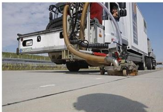
New ring road of Prague, removal concrete film, 33 cm disc
