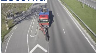
Orleans (South Paris), removal multilayer H.S.P./Paint from very soft SMA 800-1500 µ, full line
