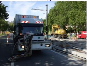
Brussel, removal Thermoplastic from SMA 1700 µ, full line
