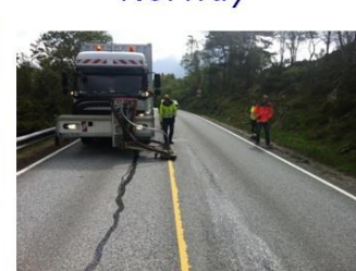
Bergen, removal Thermoplastic, full line from poor SMA, 1500 µ
