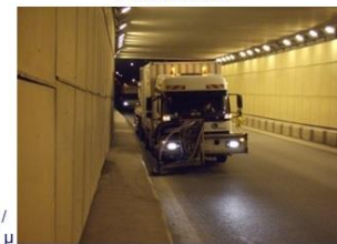
St Petersburg, removal Thermoplastic / Paint multilayer, from poor SMA, 2000 µ
