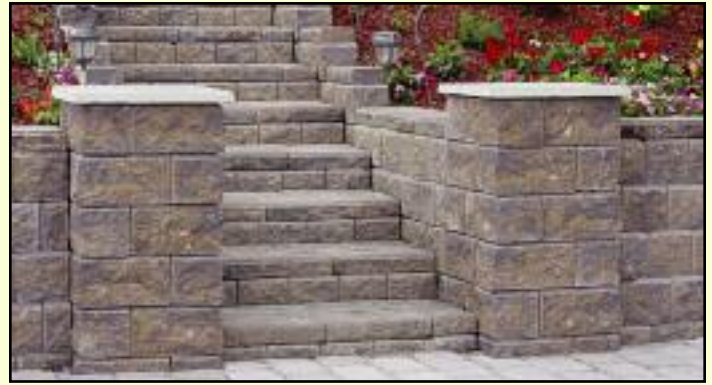
Excavate slope and place first step on compacted base
