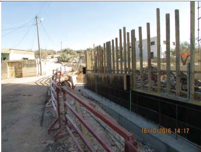
MTR-1 Concrete casting for boundary walls
