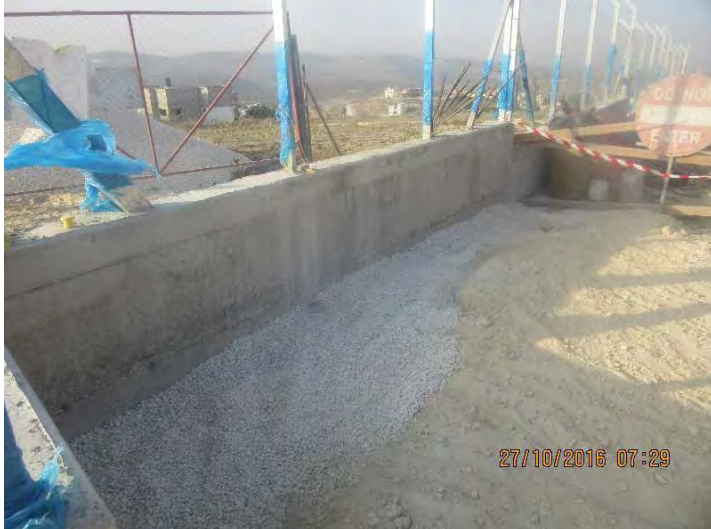
KRR-2 Cast of Concrete for Foundations of Retaining and Boundary Walls
