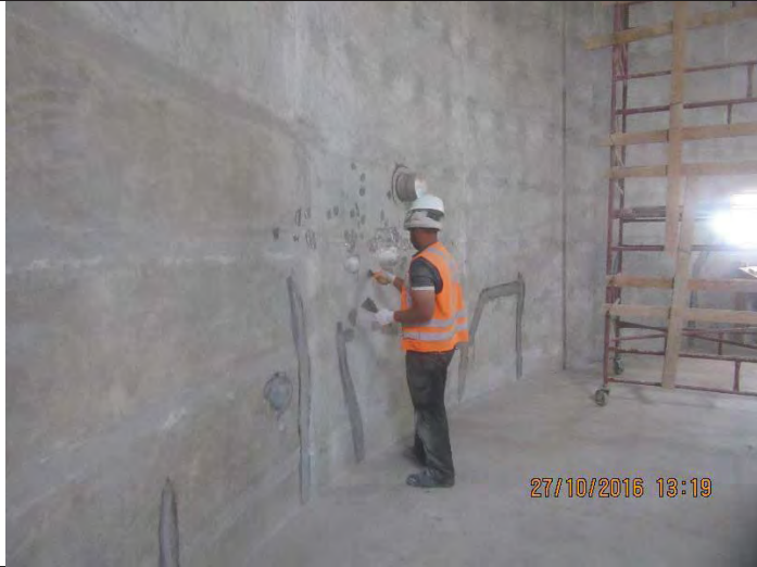
AJR-3 Repair Work for Internal Reservoir Walls
