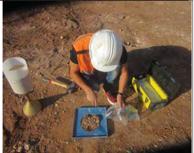
MTB-1 Compaction Test for Site Grading at MTB Yard
