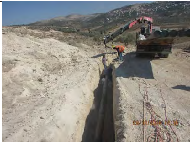
TMN-3 Installation of Anodes for CPS
