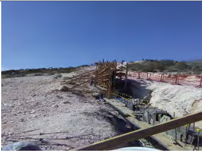
JLR-1 Formwork for Stem of Retaining Walls for Reservoir Access Road
