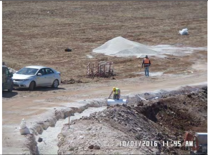
TMN -3 Pipe line works
