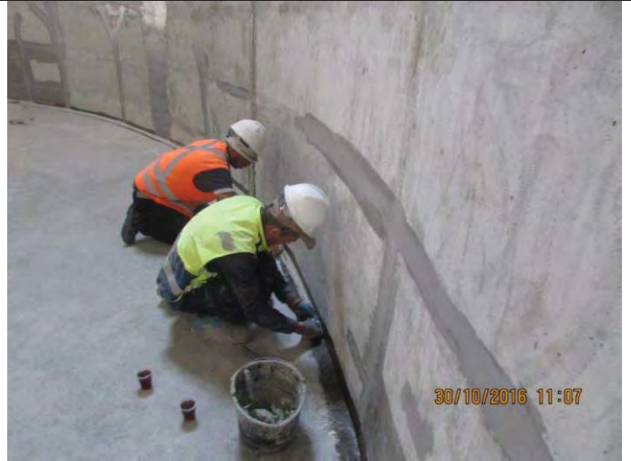
AJR-1 Internal repair in Reservoir
