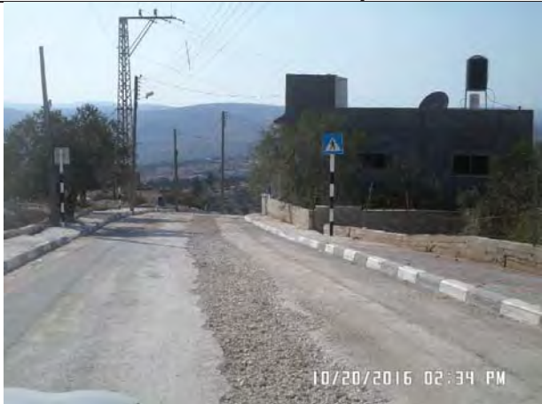
TMN-8 Excavation Works for Anodes at Cathodic Protection System
