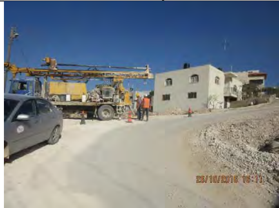
TMN-1 Installation of Anodes for Cathodic Protection System
