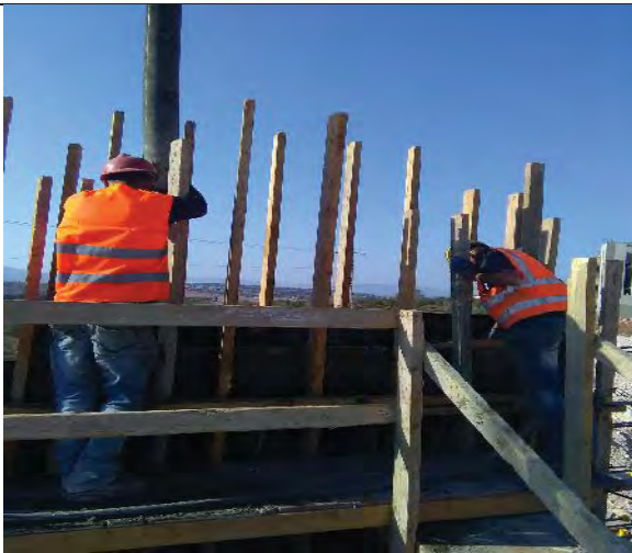
JLR-2 Casting lean concrete for RW
