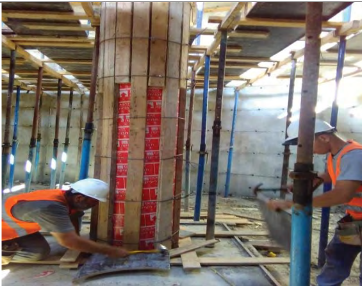
KRR-1 Reservoir's slab formwork
