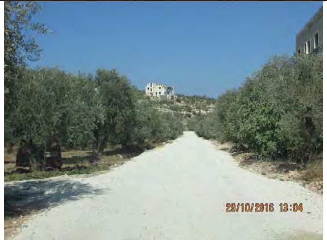
SMT-3 Spreading of Base Course Layer from STA: 1+615 to STA: 2+080
