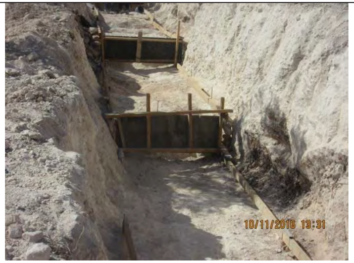
JLR-2 Duct bank works
