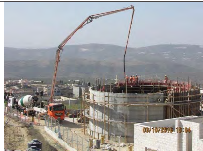
KRR-1 Reservoir walls formwork
