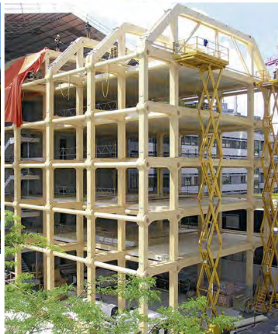
Timber frame constructions
