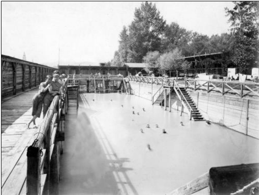
Figure 14. The Swimming Facilities in the Fabrikarm, circa 1880. Source: Unknown photographer. Schwimmschule . Photograph. 1880. Nordico Museum, Linz, Austria. Archival number: NWB-000249.
