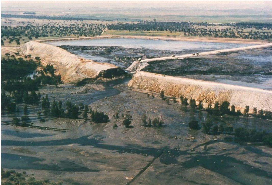
Figure 3: A view of the breached dam a few hours after the failure.
