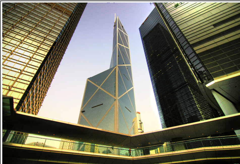
Bank of China, Hong Kong, 1989, Arch.: I.M. Pei, Ing.: Robertson, Fowler and Associates
