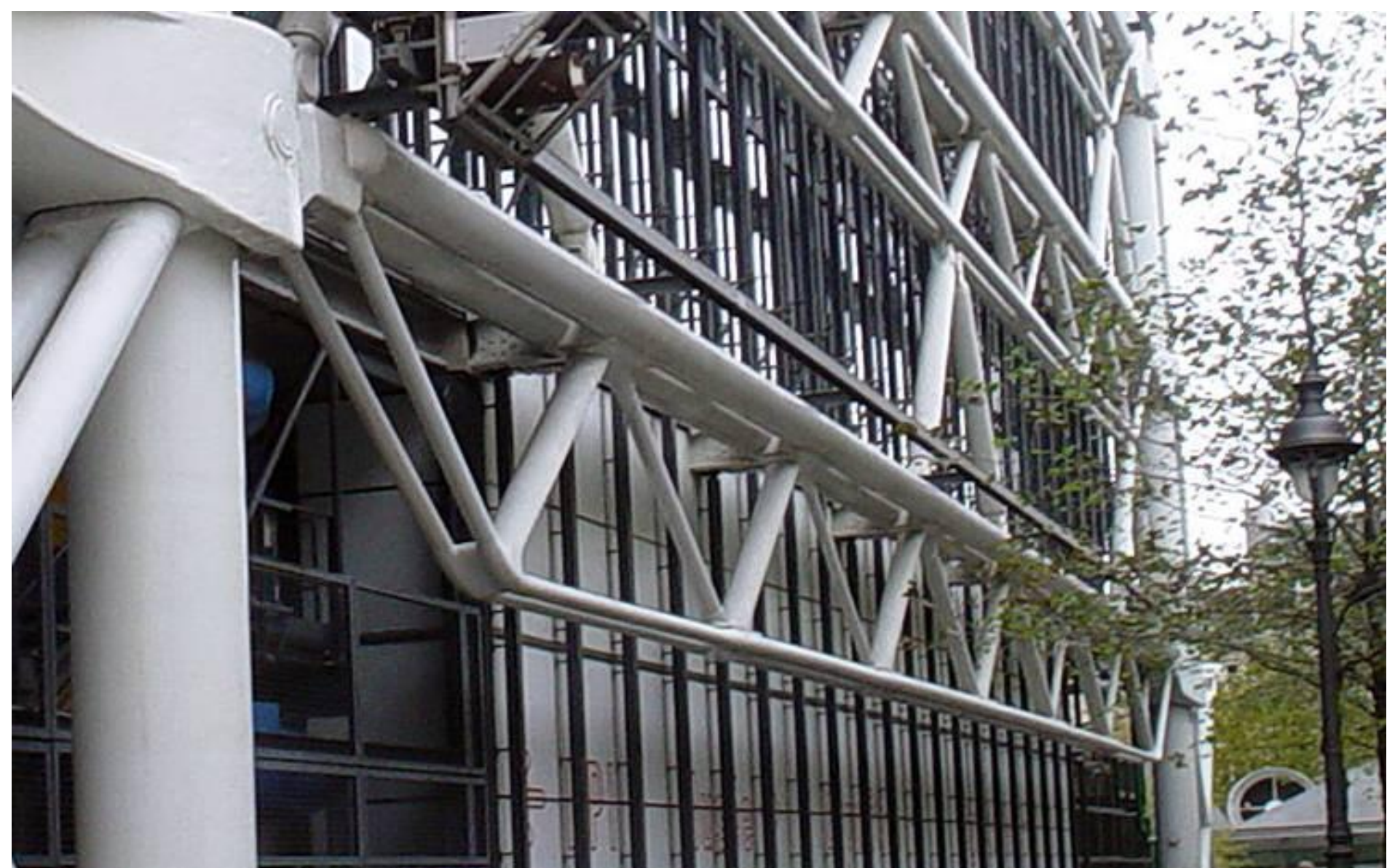
Centre Georges Pompidou, Paris, 1977, Arch: R. Piano + R. Rogers, Ing: P. Rice (Ove Arup & Partners)
