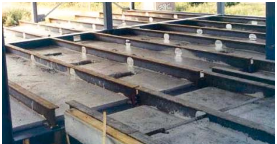
Abb. 4.7 Details des Slimline-Systems
