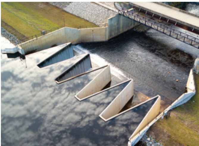
Figure 1. Hope Mills dam spillway with a 4.6 m high Labyrinth weir in North Carolina, USA (commissioned 2018). Photo courtesy of Schnabel Engineering.
