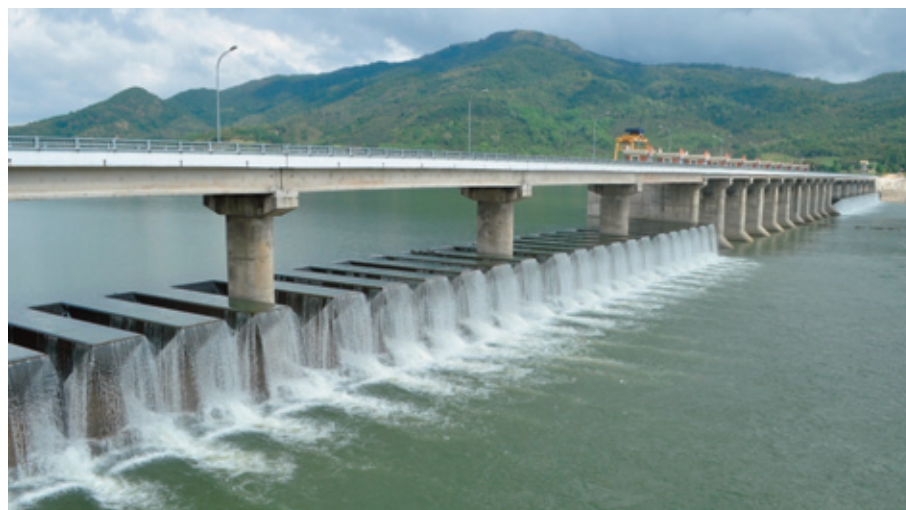
Figure 3. Van Phong dam spillway with a 5 m high type-A Piano Key weir in Vietnam (commissioned in April 2015). Photo courtesy of VNCOLD.
