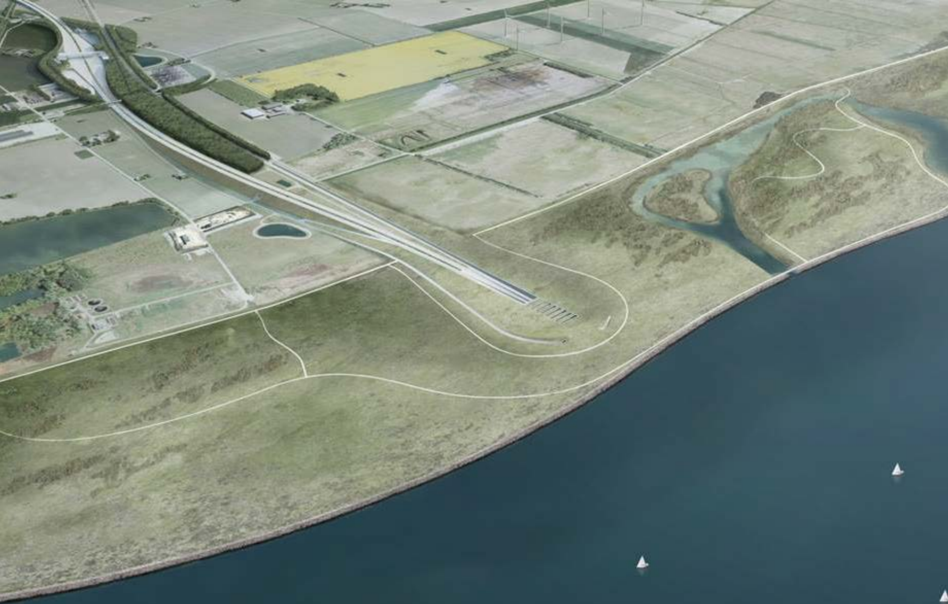
Tunnel portal on Lolland, Denmark
