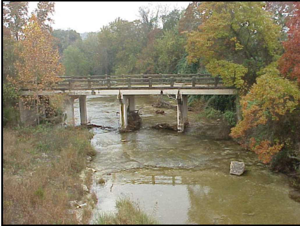
Figure 14. Old SH 27 bridge on Fessenden Branch below Fessenden Springs (11/22/00)
