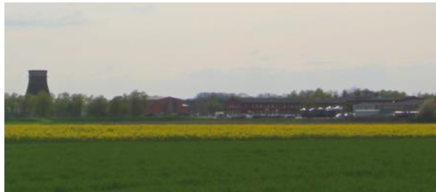
Industrial area Lüdersfeld today
