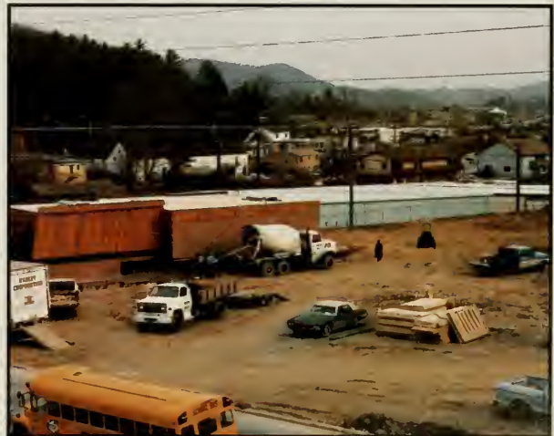
Condominiums now stand on this cleared site above Sollecito's pizza. They were constructed in a matter of days.
