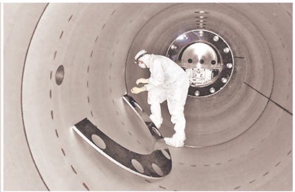
A worker installed a baffle in 2010 to control light in the Laser Interferometer Gravitational-Wave Observatory in Hanford, Wash.
