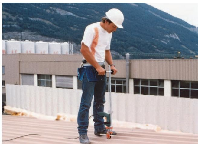
Fixing trapezoidal sheet metal using self-drilling screws
