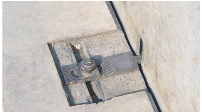
HALFEN HKZ Restraint tie with serrated washer
