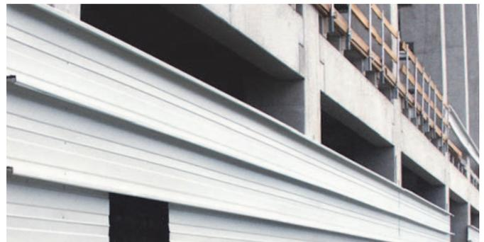
Façade fixed using HALFEN HTU Cast-in channels (Cologne Bonn Airport)
