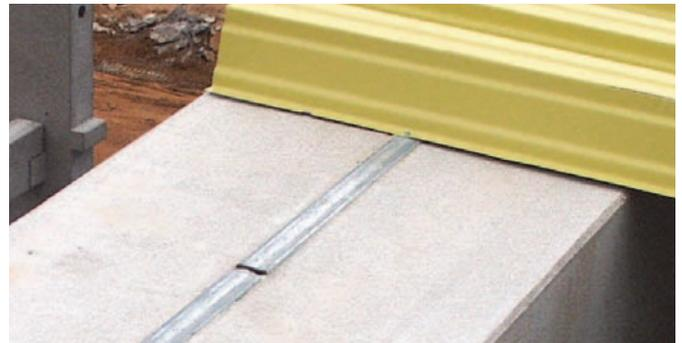
Fixing of trapezoidal sheet metal roof element
