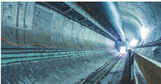
Utility fixings in TBM tunnels with curved anchor channels
