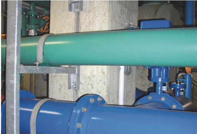
Pipe supports on vertical HZA Channels
