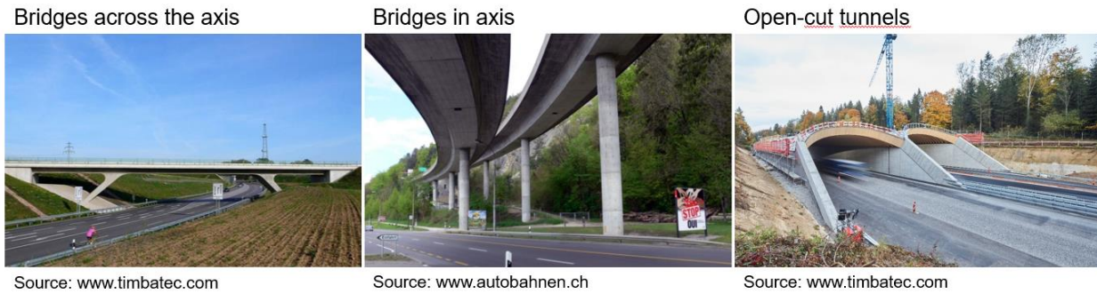
Figure 9, 10, 11: Rising demand for wood in infrastructure: Bridges across the axis, bridges in axis, open-cut tunnels
