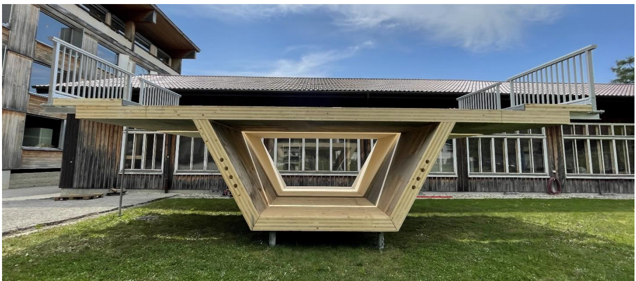
Figure 20: Box-girder modules in the courtyard of the Bern University of Applied Sciences Biel. Picture: Steffen Franke
