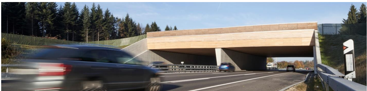
Figure 16: Built wildlife overpass Neuenkirch LU, Switzerland. Picture: Nils Sandmeier, Timbatec
