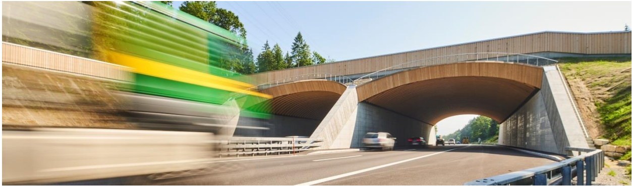
Figure 15: Built wildlife overpass Rynetel AG, Switzerland. Picture: Nils Sandmeier, Timbatec
