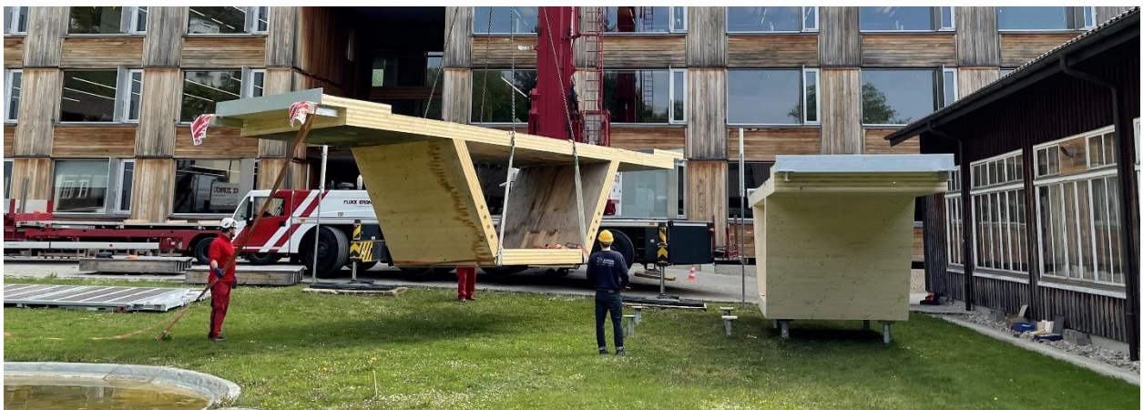
Figure 19: Installation of the box-girder modules. Picture: Steffen Franke
