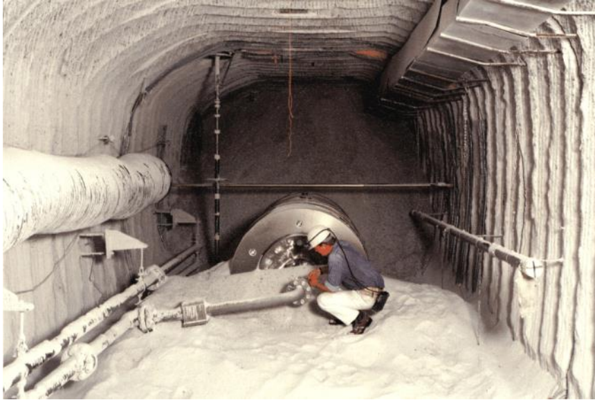
1990: Installation of test casks and monitoring system
