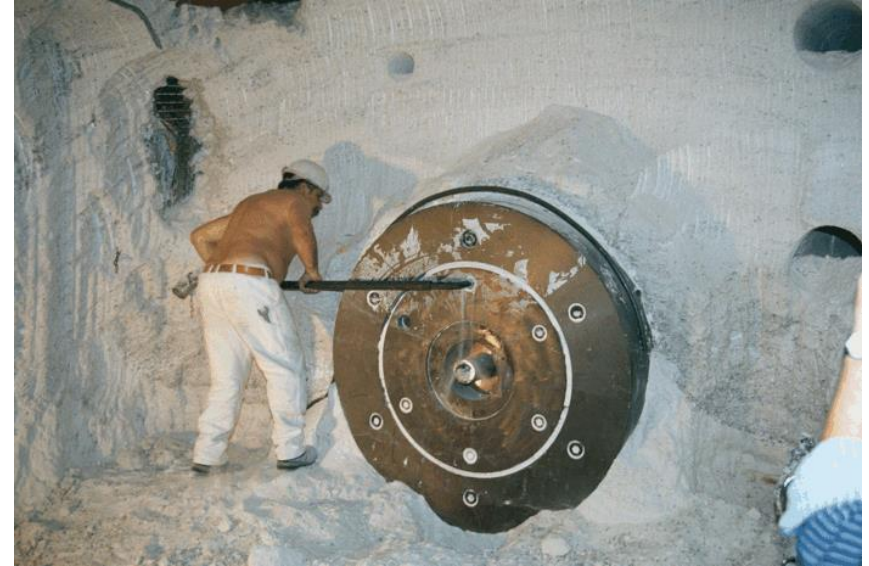
10 years later: dismantling and cask removal
