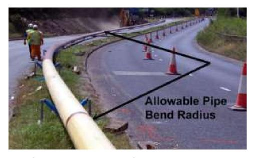
R<sub>allow</sub> → Material Bending Stress + Axial Stress due to Tension + Critical Ring Buckling
