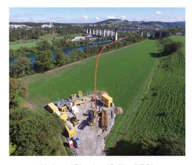
Horizontal Directional Drilling (HDD)
