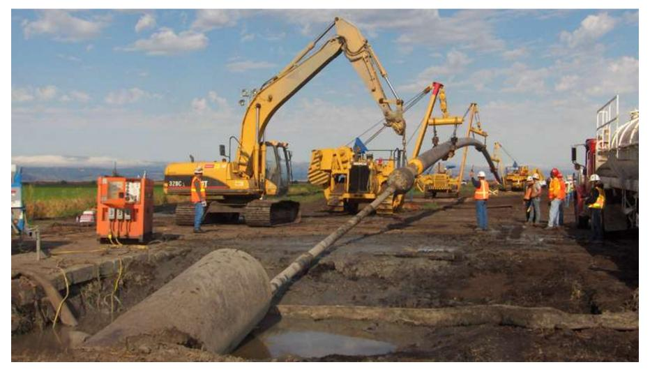
HDD Pullback Site – Large Diameter (≥ 24" OD)
