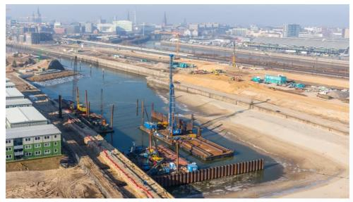
In the coming years, a sustainable "urban village" will be created around Baakenhafen harbour in the middle of the city. In the course of the redevelopment, the 340m long shore enclosure of Baakenhafen harbour had to be rebuilt as a back-anchored, heavy sheet pile wall with rising concrete spar (1.1x2.4m). Baakenhafen is located in the eastern part of HafenCity in the immediate vicinity of the Elbe bridges.
