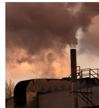
Industrial/ Commercial Processes
