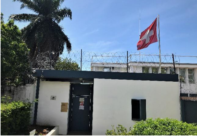
Entrance of the Embassy of Switzerland in Accra
