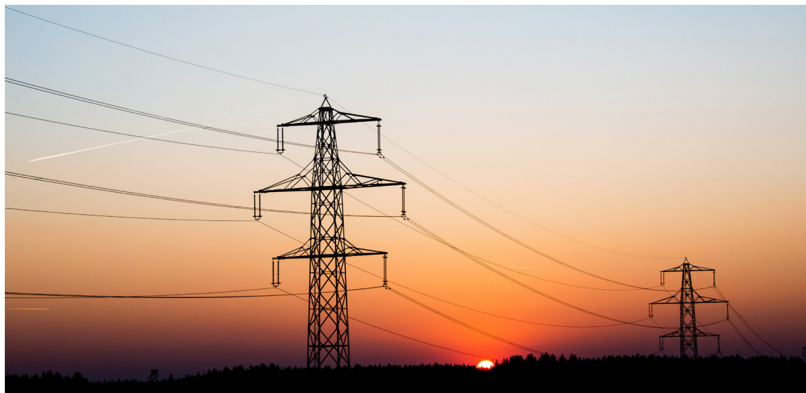
The Swiss transmission network has a length of 6700 km.
