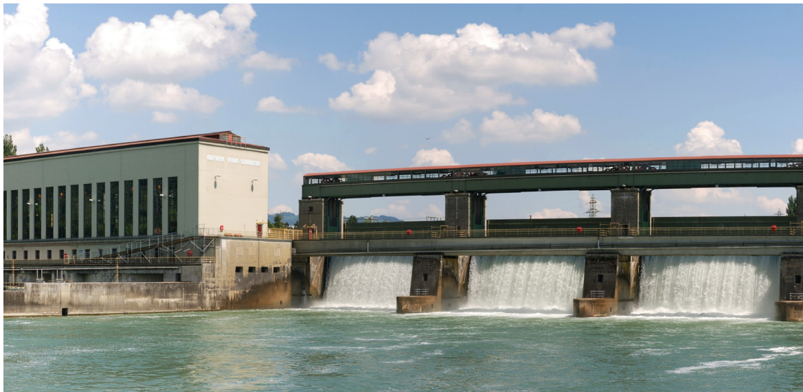
Photograph of the power plant of Ryburg-Schwörstadt 30 hydropower plants along Switzerland's borders produce electric energy.
