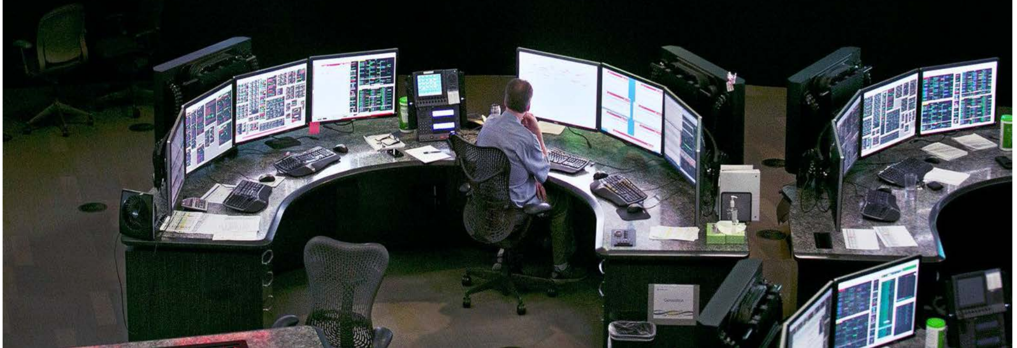
California Grid Control System The New York Times, 2018
