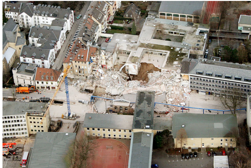
Figure 1.7: Collapse of Cologne's Municipal Archive building in March 2009 due to civil construction (drilling) for the new subway line [32]
