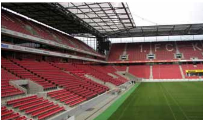
Fixing of safety rails, Rheinenergiestadion Cologne
