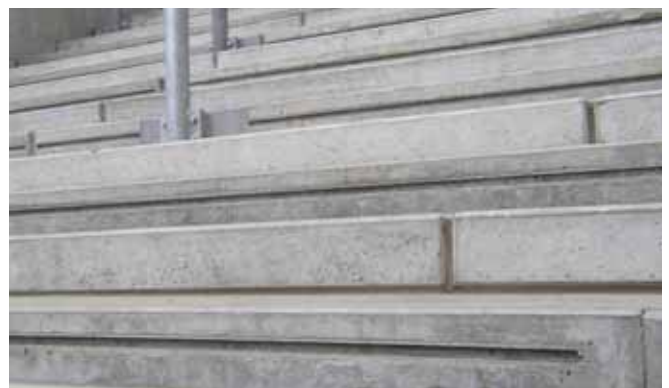
Fixing of safety rails, Rheinenergiestadion Cologne
