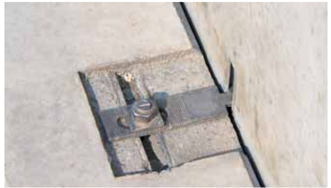
HALFEN HKZ Restraint tie with serrated washer
