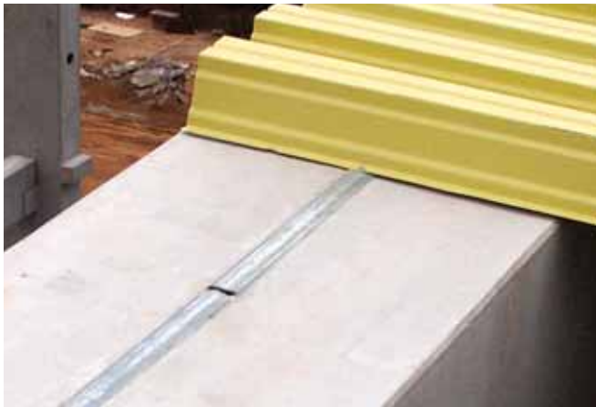
Trapezoidal roof sheet metal attachment
