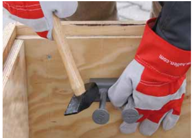
Nail the HALFEN Cast-in channel to the formwork
