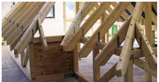
Timber pitched roof construction
