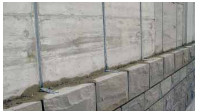
HALFEN ML Brick-ties anchor system
