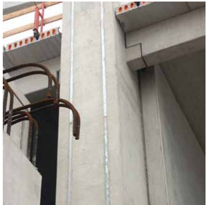
Vertical HALFEN HTU Cast-in channels for connecting façade panels
