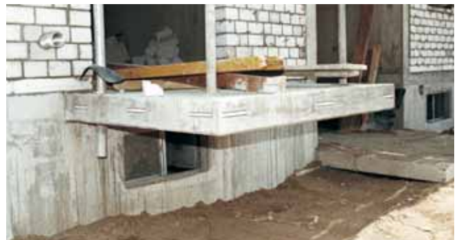
Cast-in HGB Channel, residential building
