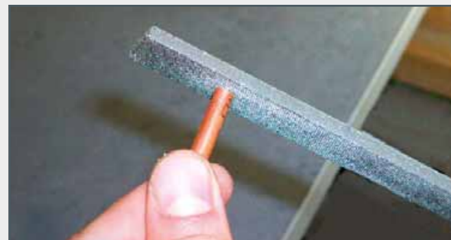
Filing the saw cut smooth, the cutting surface must be perpendicular to the pipe axis
