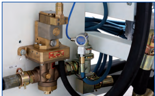
Electronically controlled fresh water valve
