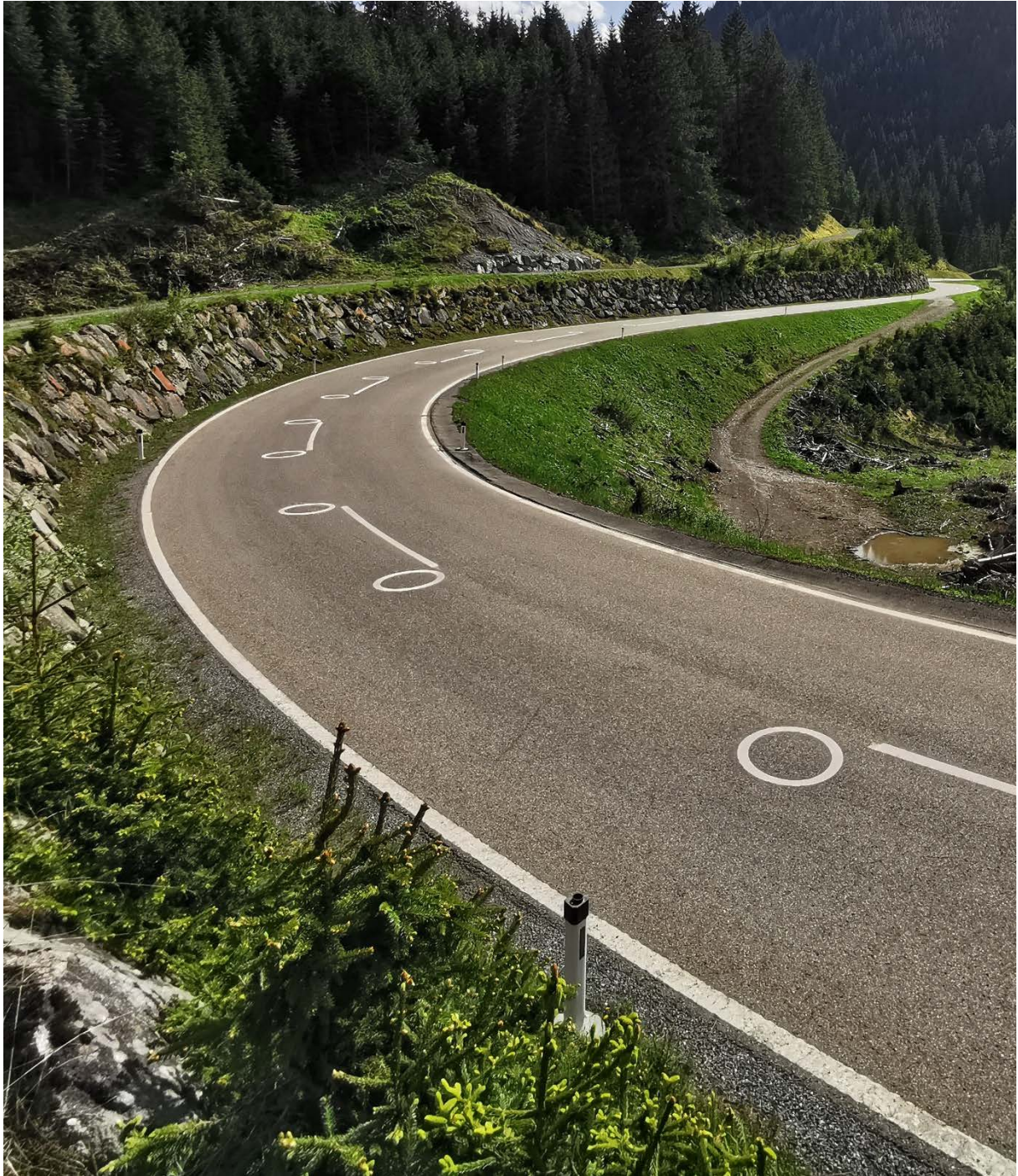
Figure 3: Ellipse markings in the Namlos Valley
