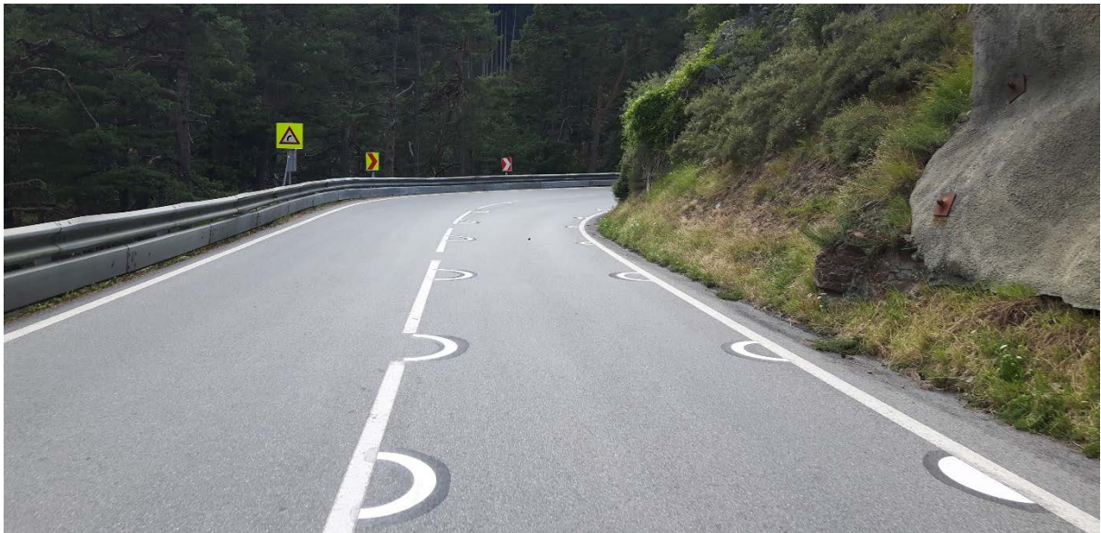
Figure 17: Road markings on a right-hand bend
