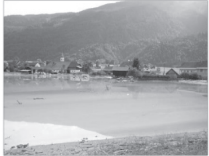
Abb. 6: HW2003, Rückstau hinter Gaildamm Fig. 6: flood 2003, backwater behind the dam
