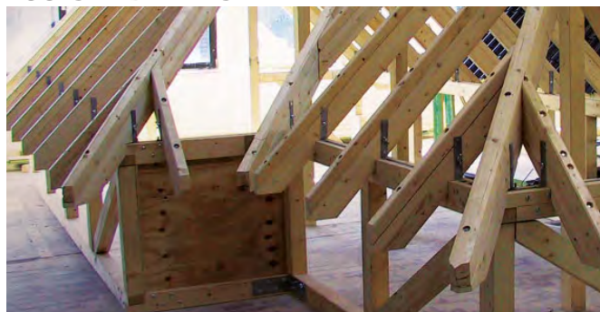
Timber pitched-roof construction
