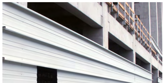
Façade fixed using HALFEN HTU Cast-in channels (Cologne Bonn Airport)
