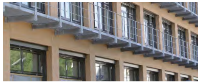
Fixings for emergency access balconies (Vertical installation of HALFEN Channels)
