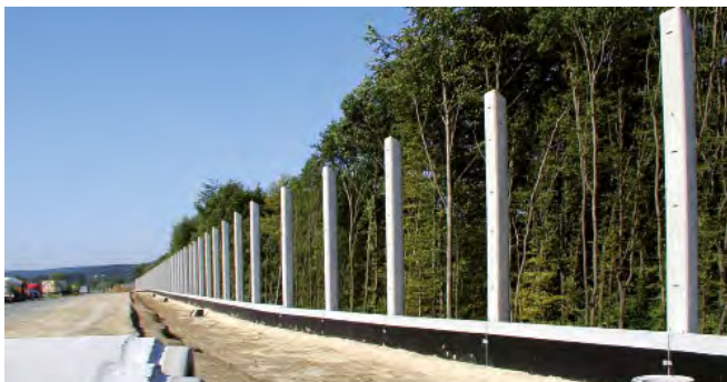
Fixings of noise barriers to concrete posts
