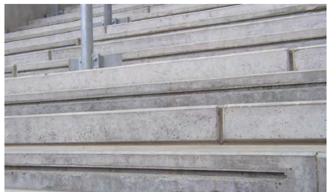
Fixing of safety rails, Rheinenergiestadion Cologne
