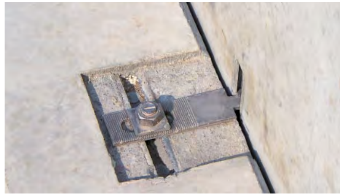
HALFEN HKZ Restraint tie with serrated washer
