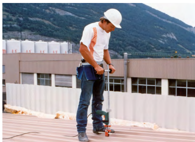
Fixing trapezoidal sheet metal using self-drilling screws
