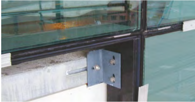
Fixings for curtain wall façades
