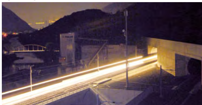
Lötschberg-Base tunnel, Switzerland
