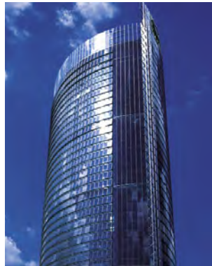
Post office Tower, Bonn
