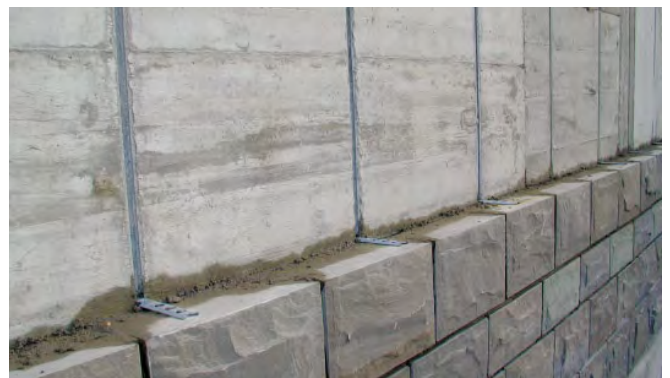
HALFEN ML Brick-tie anchor system
