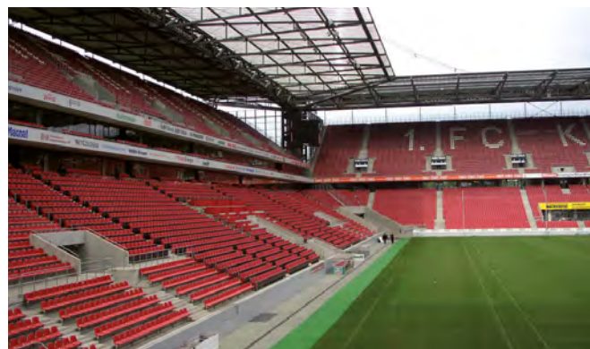
Fixing of safety rails, Rheinenergiestadion Cologne
