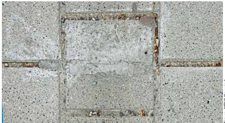
Fig. 24: Jointing mortar of a substandard quality
