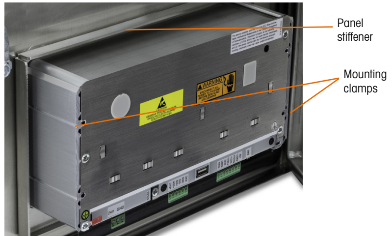
Figure 2-6: Panel Stiffener Bracket Installed
