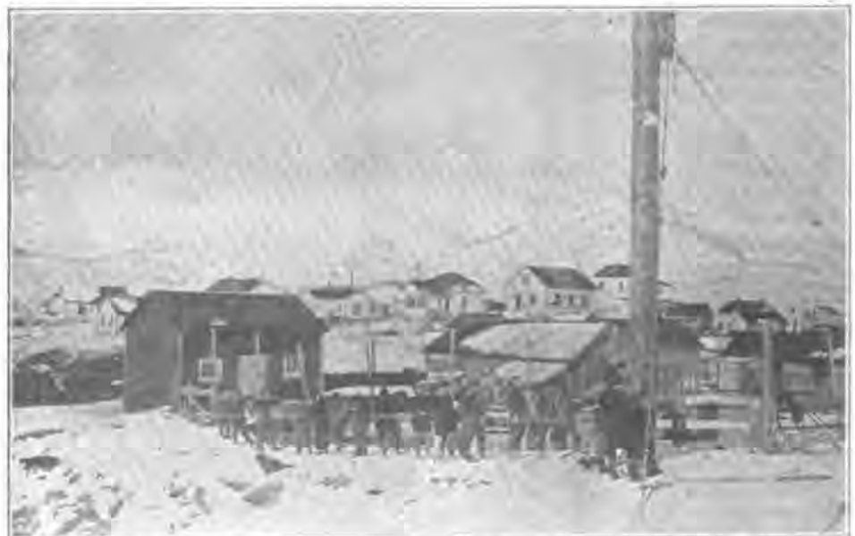
Raising wireless masts in Alaska is a cold job. Here the rigging gang are hard at it, sending up a topmast.
