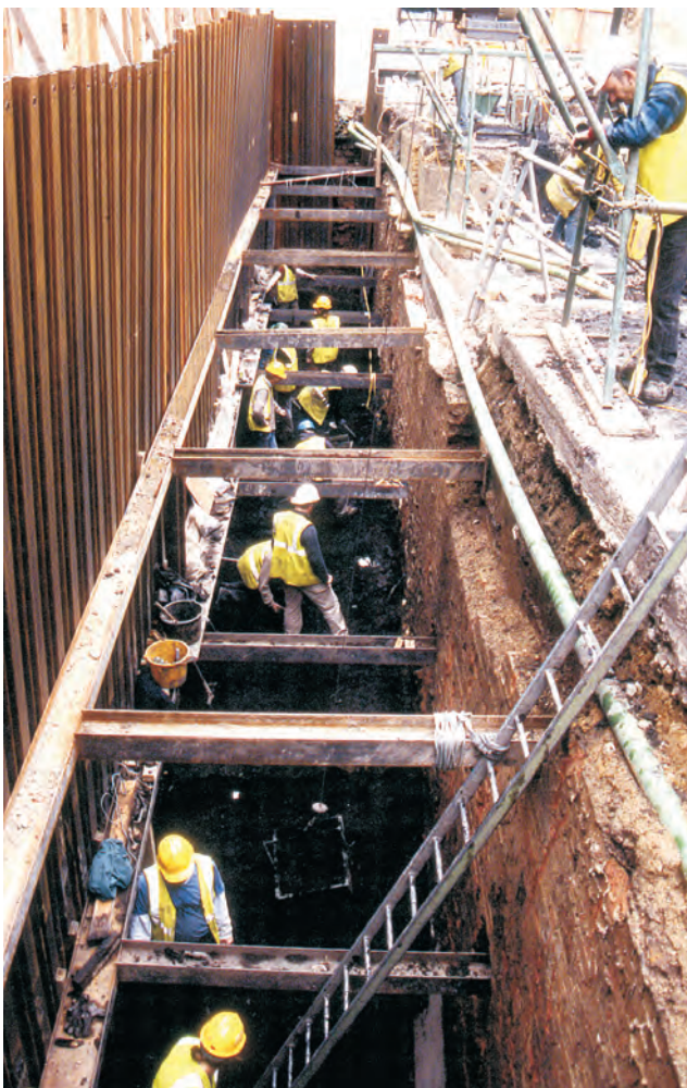
Fig. 4 Area 3 during excavation, looking south
