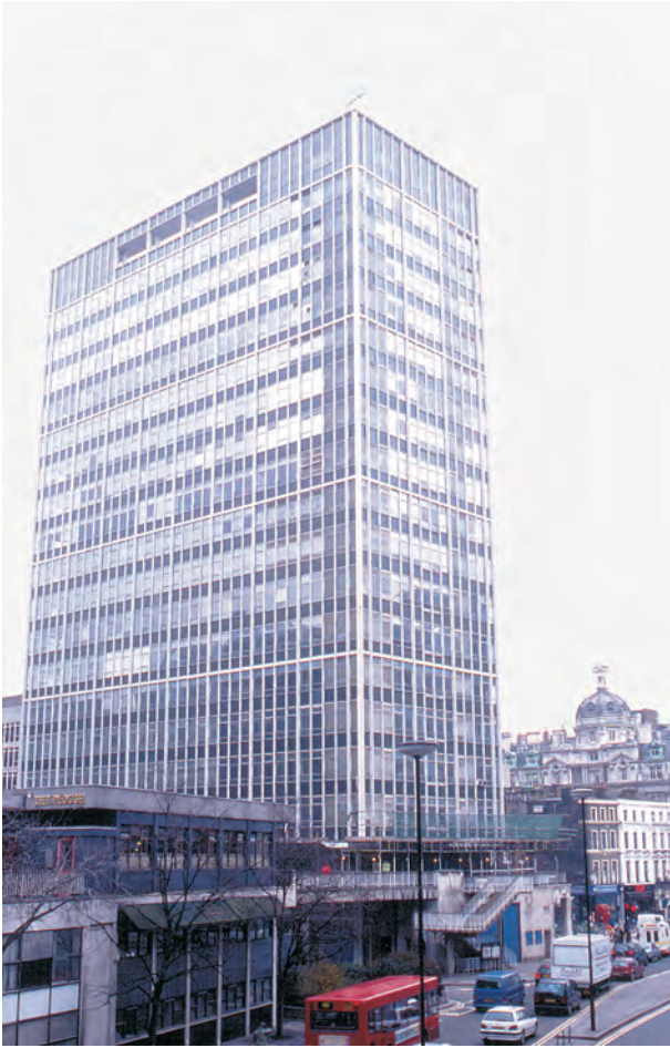
Fig. 2 Moor House tower, before redevelopment, looking northeast
