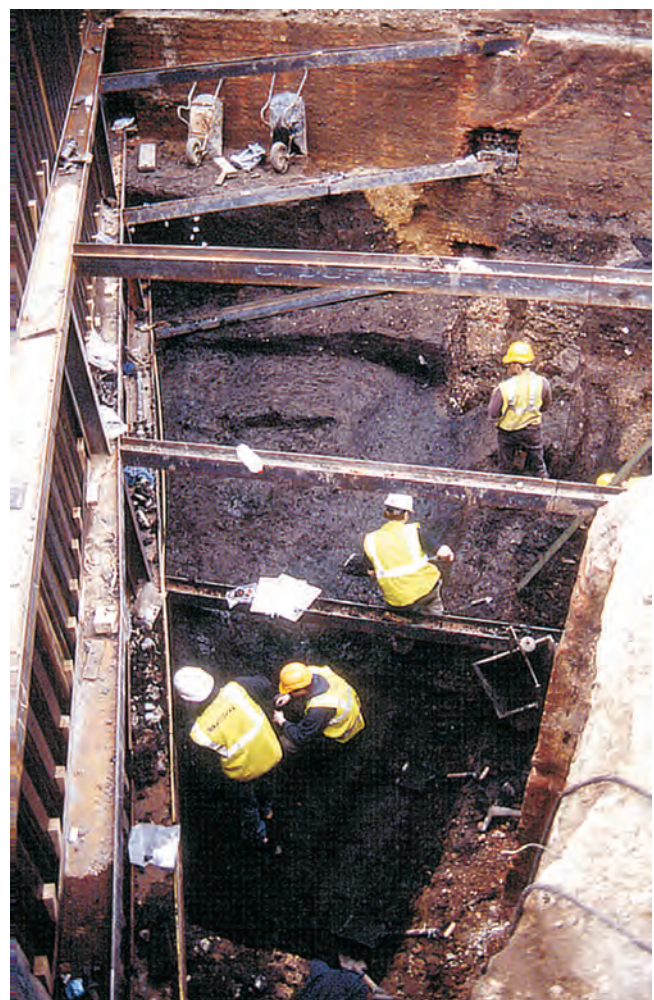
Fig. 6 Area 2 during excavation, looking west
