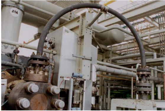
Fig.4.2.2 Detail of layout for hypercompressor suction piping
