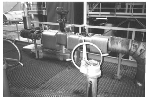
Figure 6: Photograph of the bypass section
