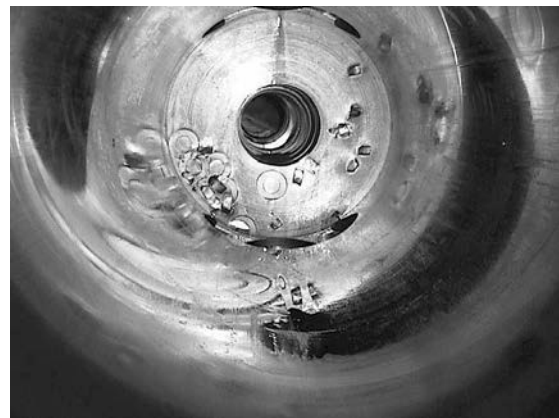
Picture 4: Cylinder showing signs of valve debris attack.
