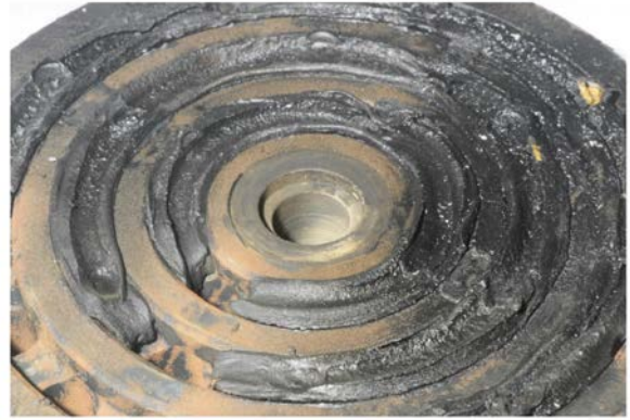
Fig: 8 – Ring Valve Failure
